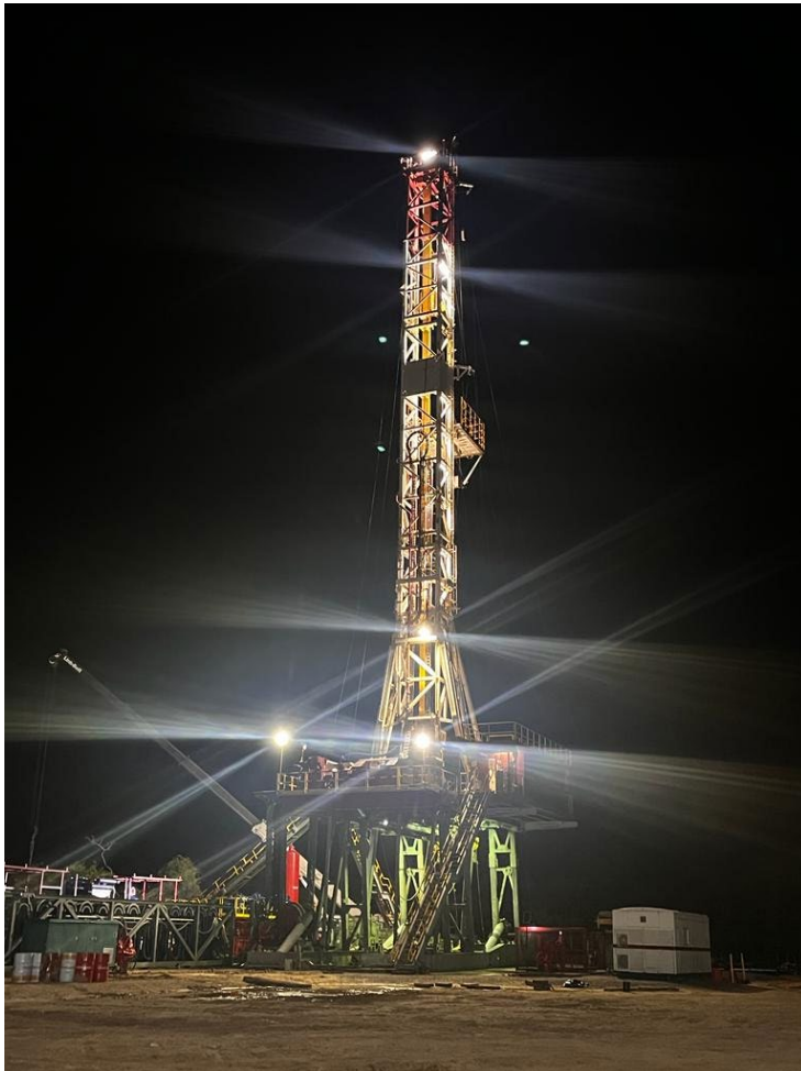
Drilling Rig at Aruchara-3 Platform
